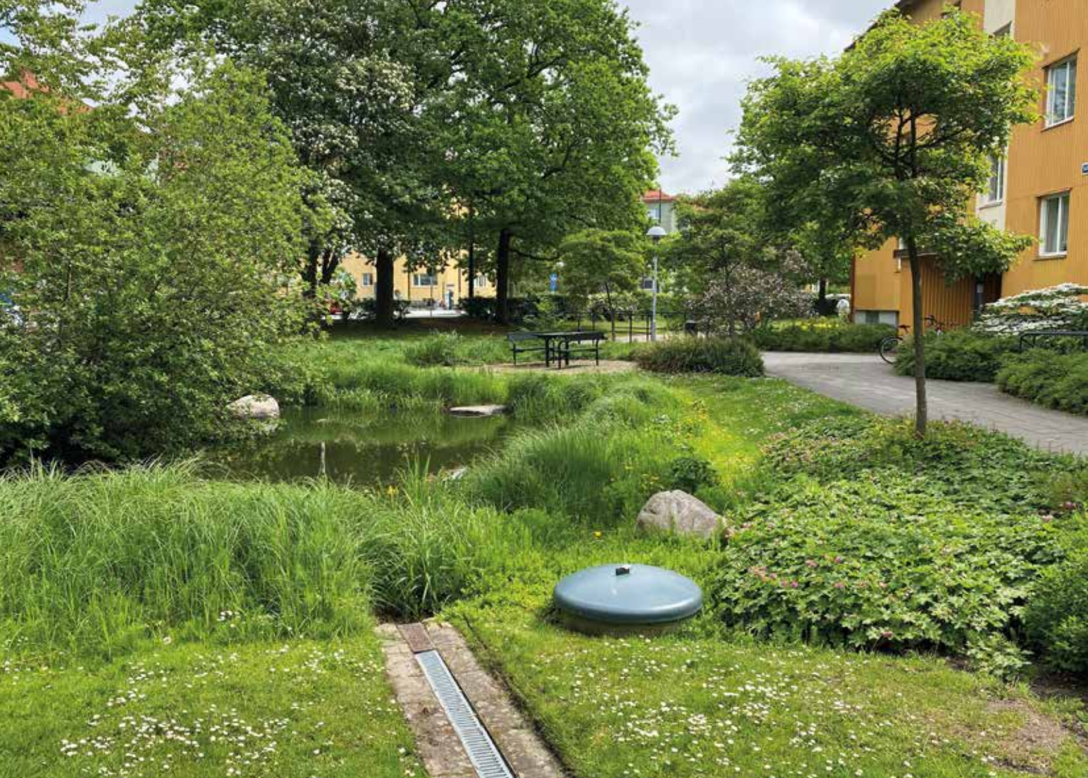
Example of climate adaptation with blue-green solutions in Augustenborg in Malmö. In areas where properties were often impacted by flooding in the past, drainage systems have been built that include water channels and retention ponds.
