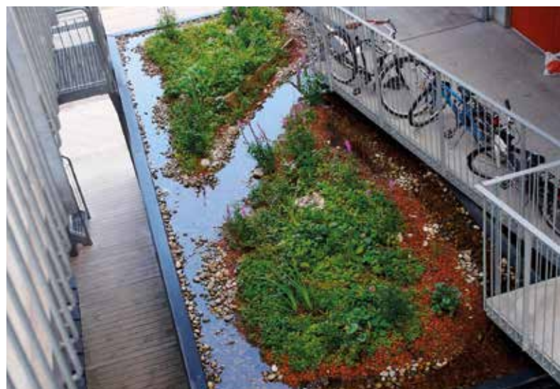
Blue-green systems provide a buffer for rainwater and reduce the risk of flooding.
